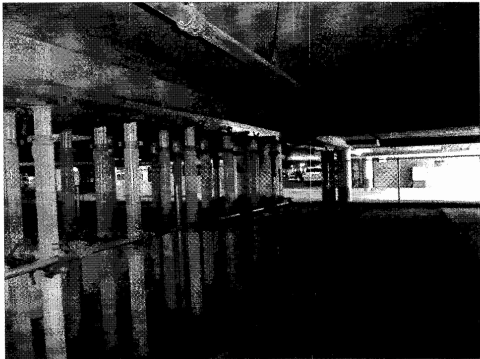
Photo 3: Existing Shoring Along Expansion Joint
