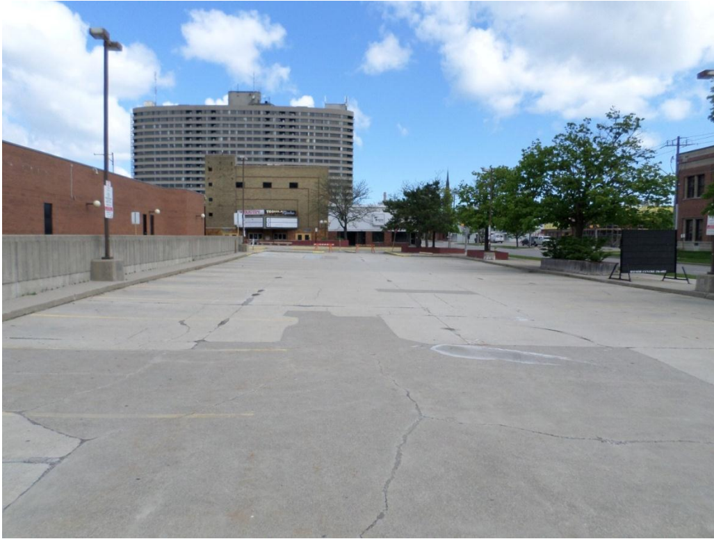
Photo 1: Parking Garage Roof Deck at Bayside Mall
