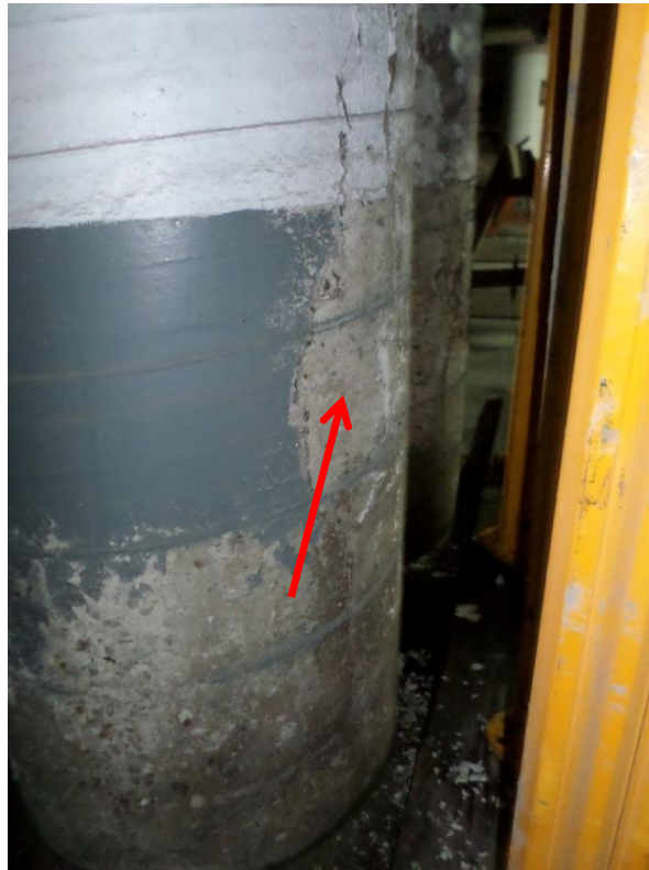
Photo 5: Column Concrete Deterioration Caused by Leakage Through the Expansion Joint
