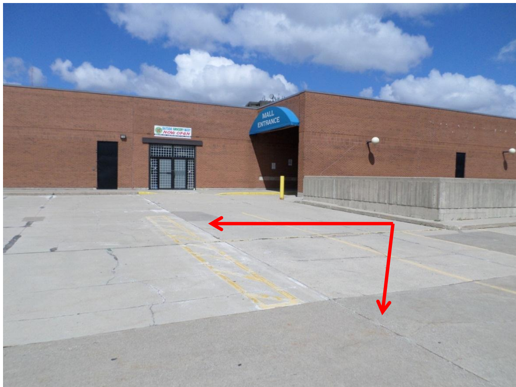
Photo 2: Location of Garage Roof Deck Expansion Joint (red arrows).
