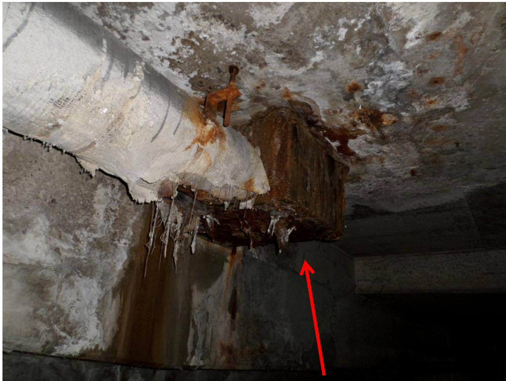
Photo 6: Typical Corrosion Deterioration at Garage Roof Slab Drain
