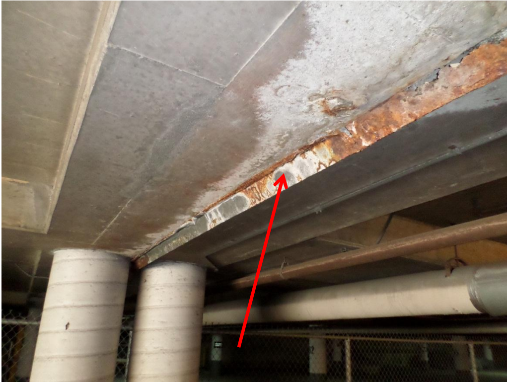
Photo 3: Leaking Expansion Joint From Garage Roof Slab Underside
