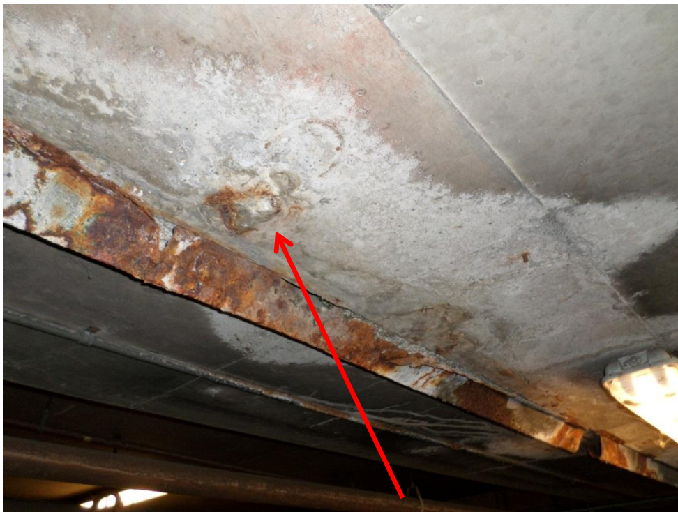
Photo 4: Concrete Deterioration Caused by Leakage Through the Expansion Joint
