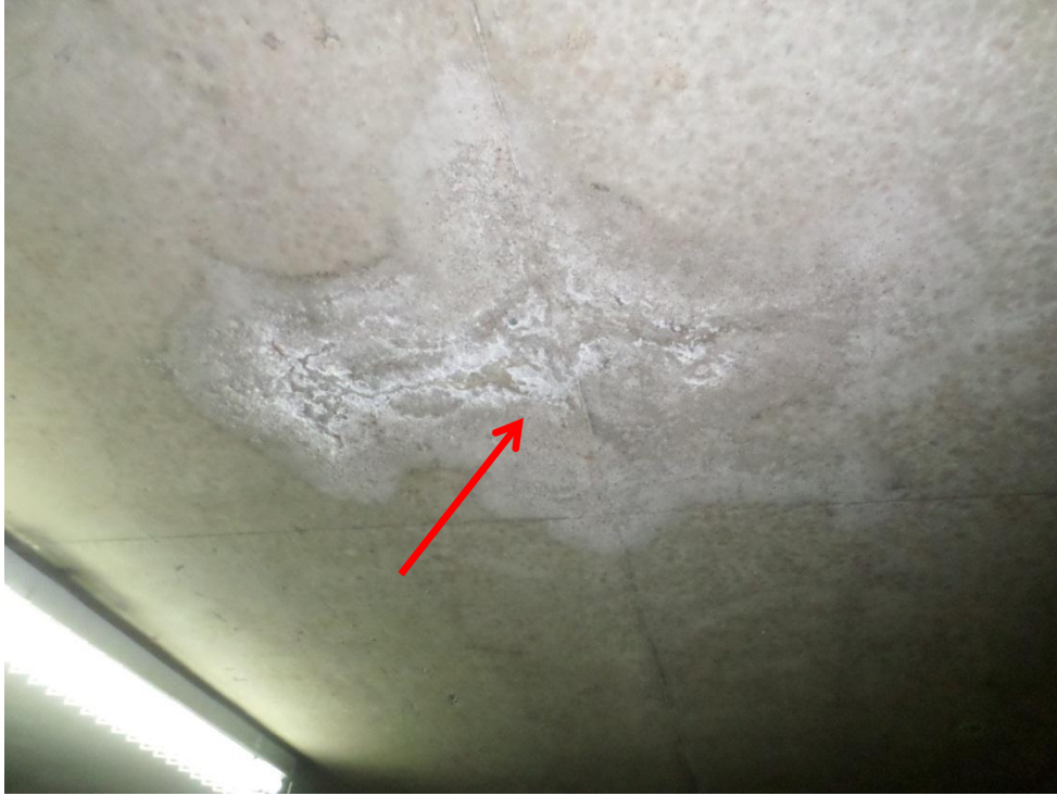
Photo 7: Staining and Deterioration Caused by Localized Garage Roof Slab Leakage
