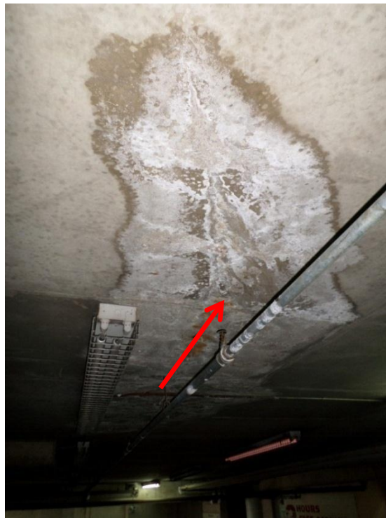
Photo 8: Staining and Deterioration Caused by Localized Roof Slab Leakage
